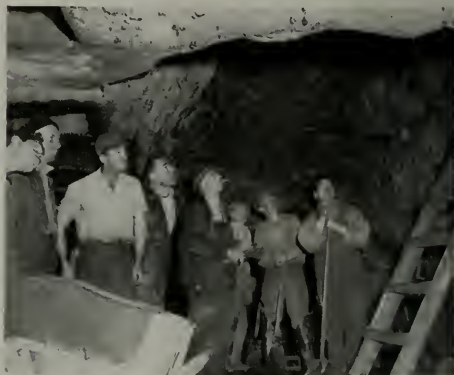
The above photograph taken at Bethlehem's San Francisco yard, shows a hole 20 feet long by 12 inches wide on the starboard side forward in the bottom of the SS Sea Satyr, C-3 freighter built by Ingalls in 1945, now owned by American Mail Line. Damage was caused by a contact mine as the vessel was backing into anchorage at the Celebes Islands, damaging over 50 per cent of the ship's bottom. Accommodations for 12 passengers will be added.
